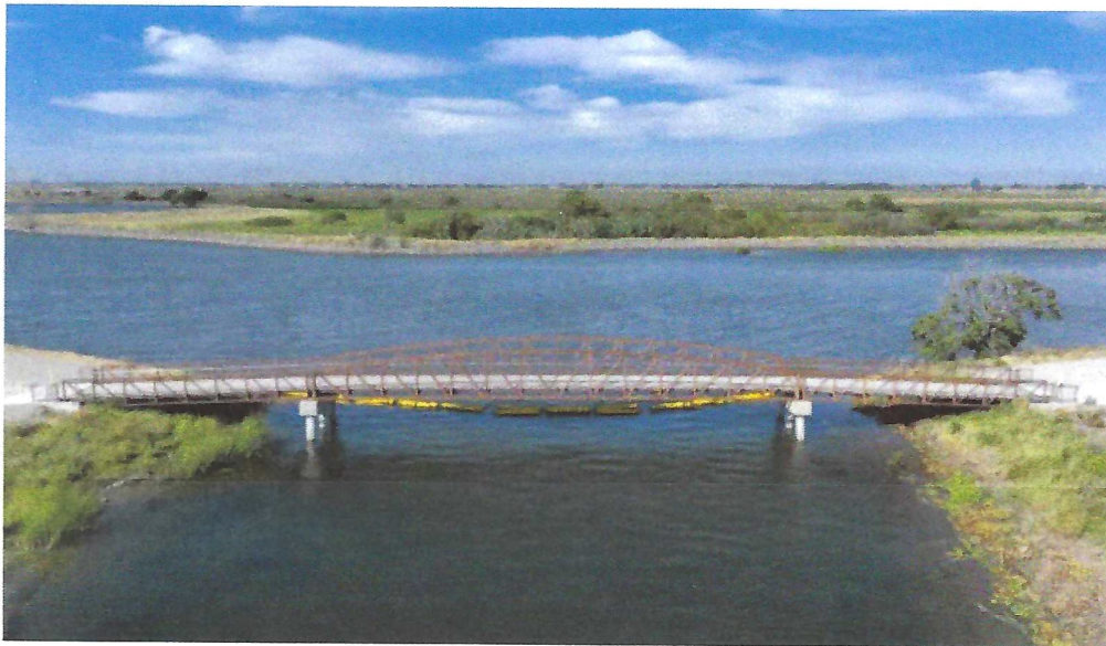
A drone view of a new pedestrian and bicycle bridge over Marsh Creek as it meets Dutch Slough in Oakley, Calif., on Tuesday, August 1, 2023. (Jane Tyska/Bay Area News Group)
